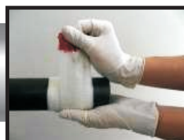
APPLY PIPEFIX TO PIPE
